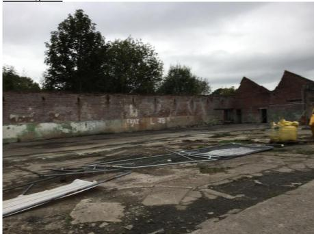
The proposal is to re-use some of the remaining lower brick walls on all sides of the structure and erect a new industrial building that would occupy the footprint of the former building and measure 46.6m long x 12.6m wide. It would extend up to 7.0m to the ridge of a shallow pitched roof. The proposed building would be divided into six units, five of which would be similarly sized (70sqm) and the sixth would be larger (181sqm).
